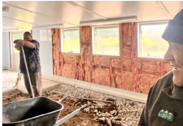
Builder Arron Whatuira & Guy Te Kahika removing floor.
